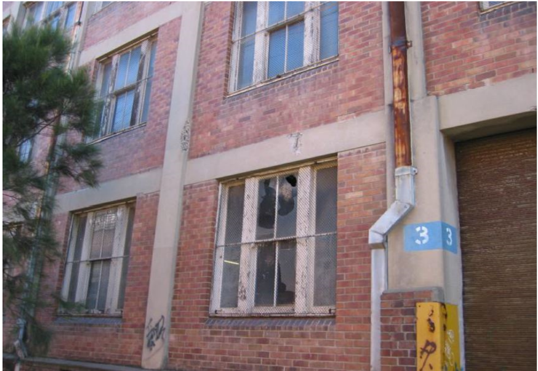
Figure 6 Typical deteriorated façade of the AML&F Woolstore building (Source: EJE Heritage Management Guidelines, Wickham Woolstores)
